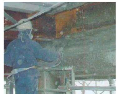
喷涂式岩棉 (生锈后脱落)
