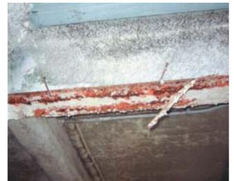
喷涂式岩棉 (生锈后脱落)
